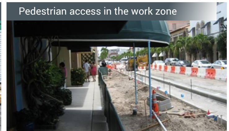
Temporary walkways installed
